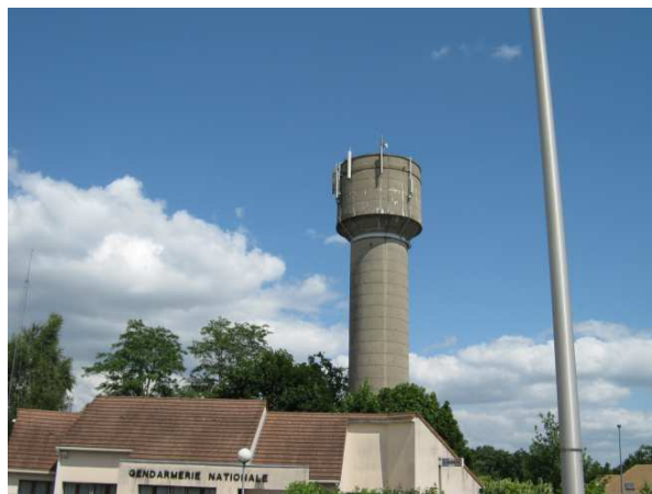
Figure 2 . Station de base 2
